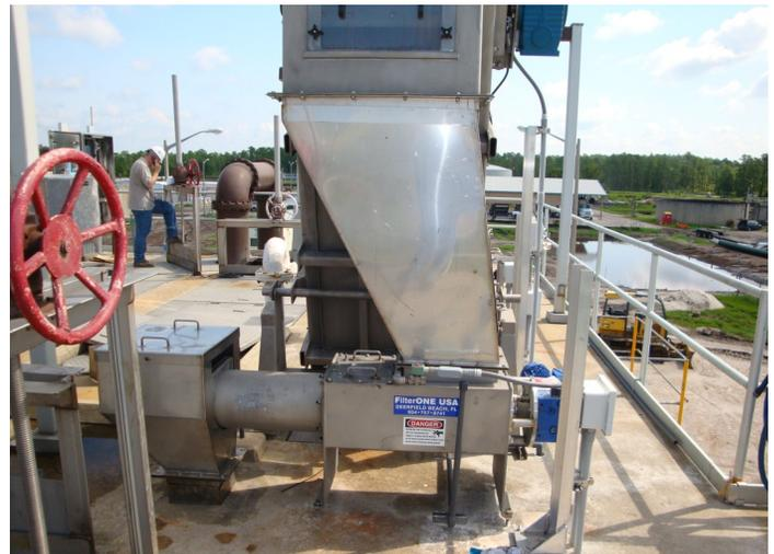
The wet solids that enter the F-1 Compactor are discharged with a reduction in water content of at least 80 percent.
